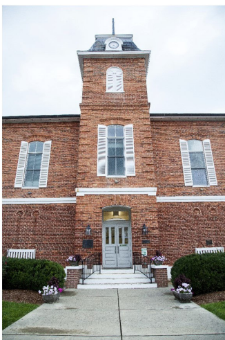
Transylvania County Courthouse, built in 1874-1950
