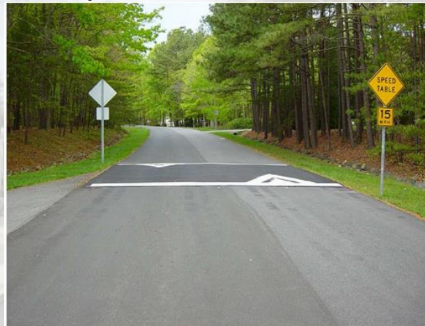
Figure 3.12.1. Typical Speed Table Application
