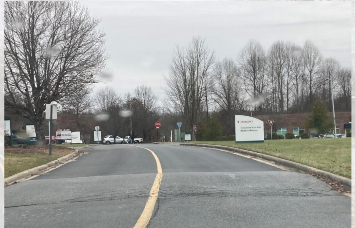
Speed table/hump at entrance to TRH Emergency Unit
