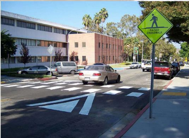
Figure 3.14.2. Typical Raised Crosswalk Application
