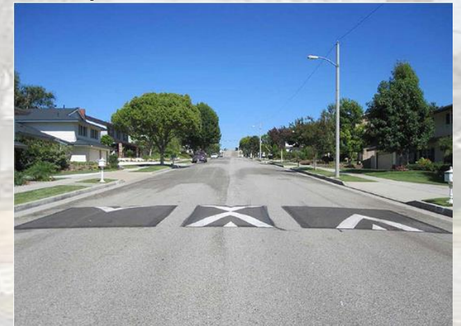
Figure 3.11.1. Speed Cushion with Passage that Straddles Centerline
