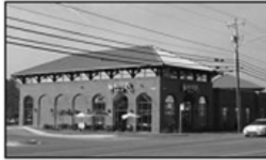
FIGURE 5.4B: EXAMPLE OF PITCHED ROOFS WITH EAVES
