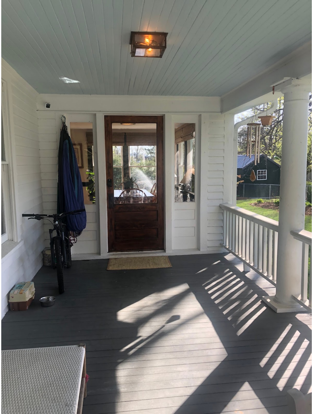
12. Secondary Entrance on South Elevation
