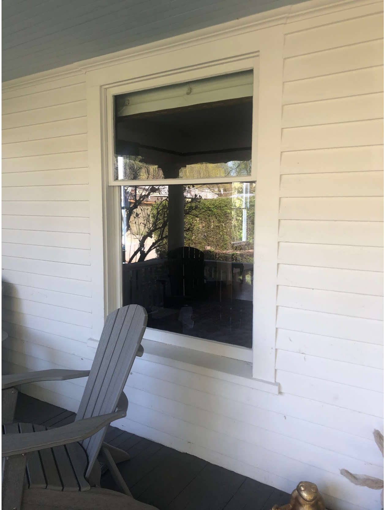
11. Window on Front Elevation
