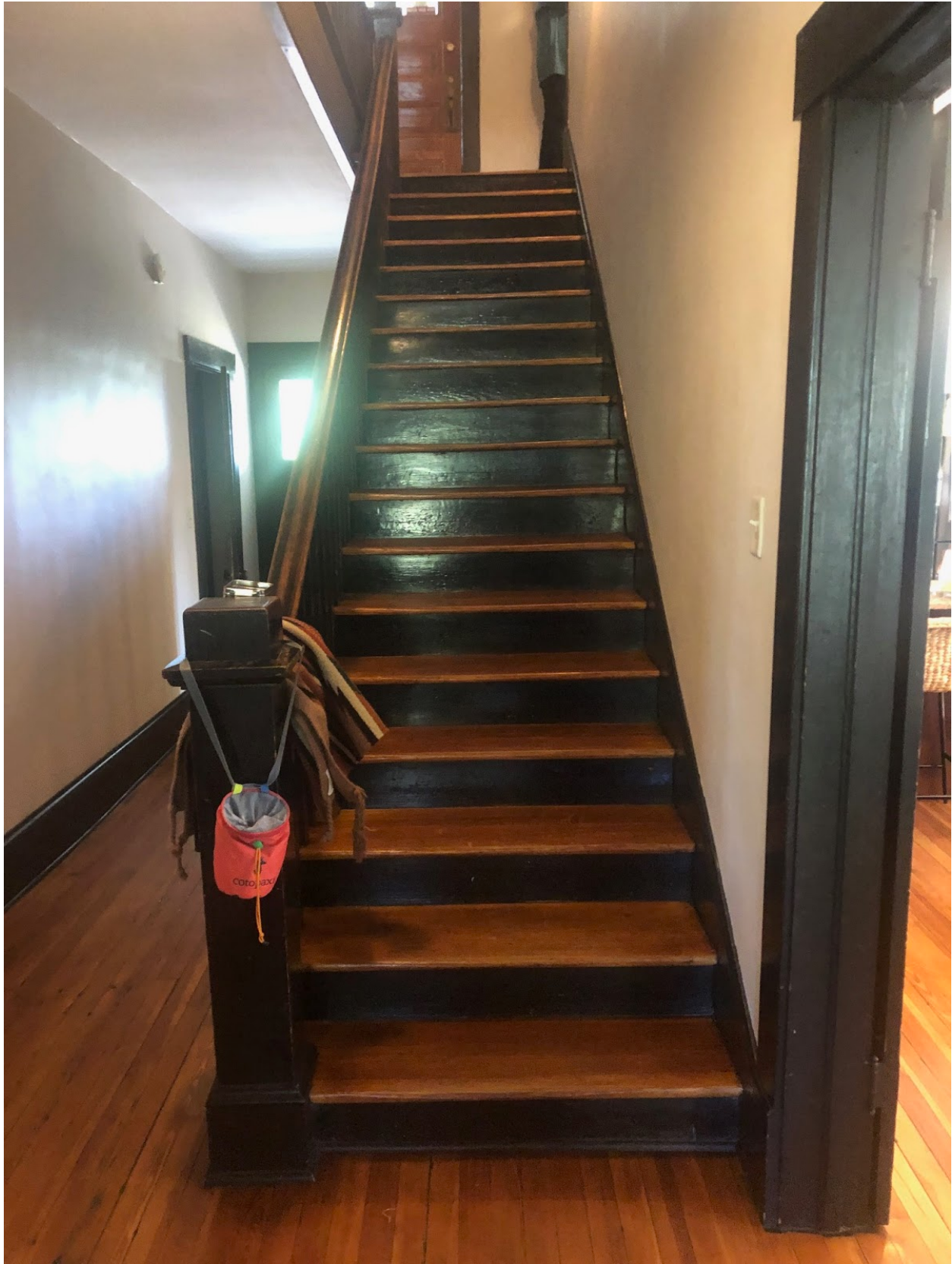
21. First Floor Staircase
