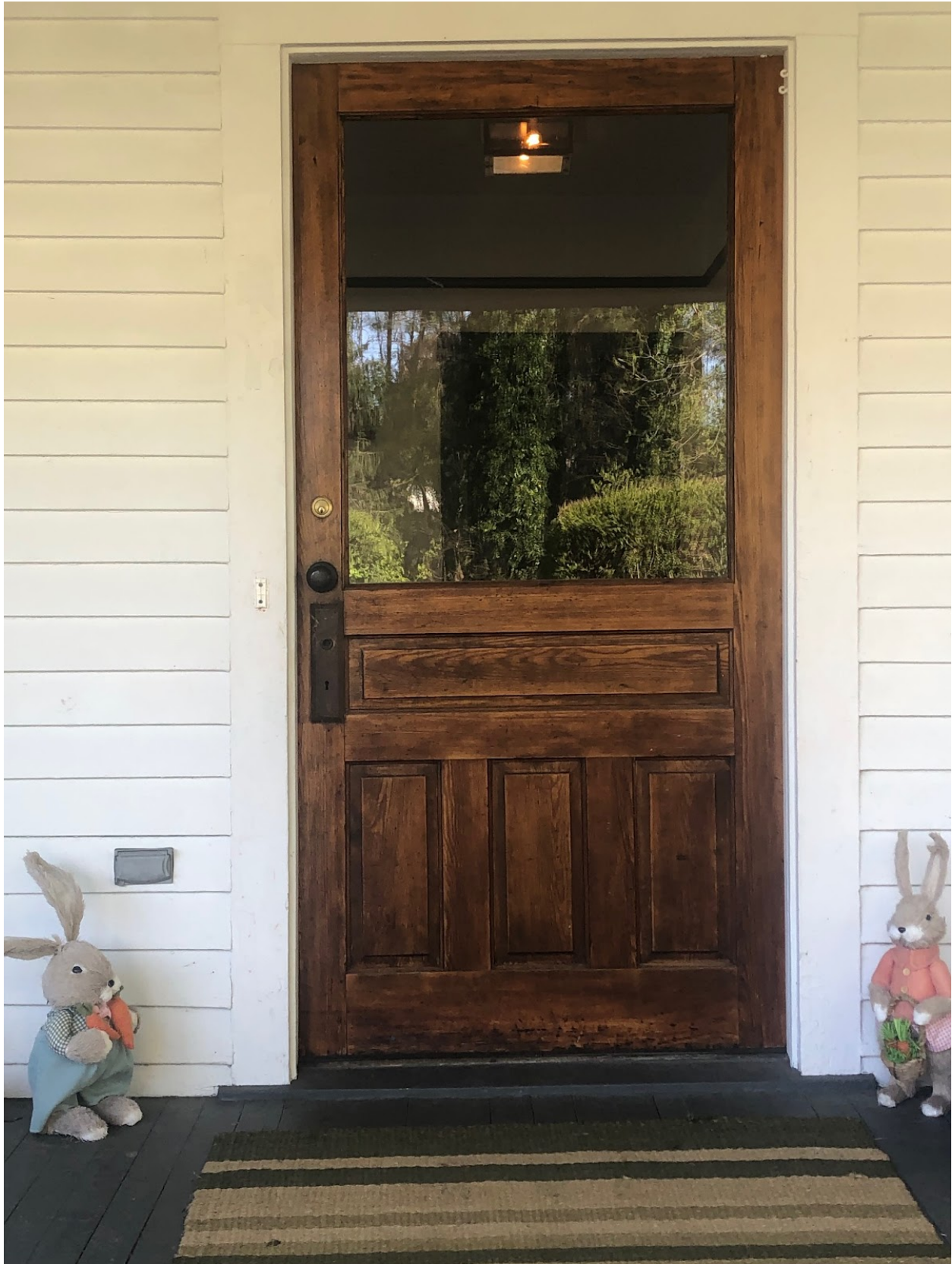
10. Primary Entrance on Front Elevation
