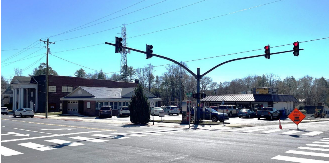
8. Context – South Corner of Main and Johnson Streets
