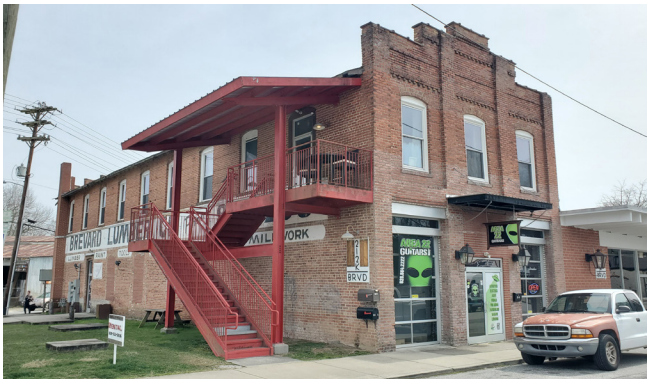
Image 48. Brevard Lumber Company, Lumberyard District.
