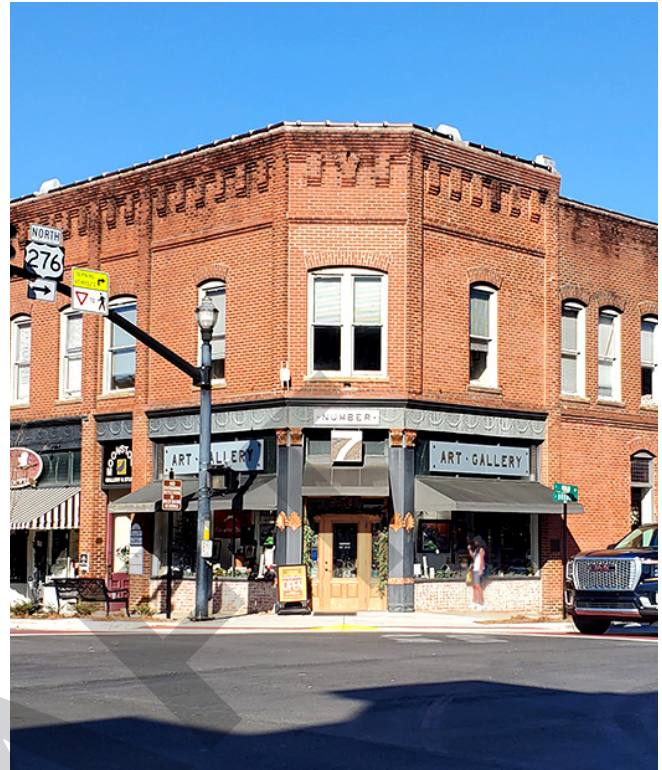
Image 88. McMinn Building on Main Street, Downtown Brevard.
