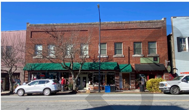
Image 49. The Pickelsimer Building in Downtown.
