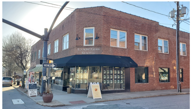
Image 46. Brick masonry vernacular building in Downtown.
