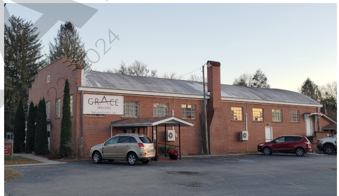
Image 76. American Legion building, 115 East Morgan Street.
