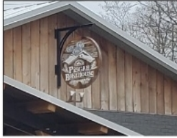
Unpainted vertical plank siding
