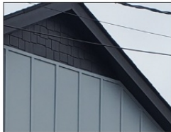
Painted fiber cement board and batten siding
