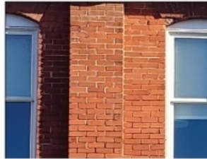
Red brick wall with a structural pilaster
