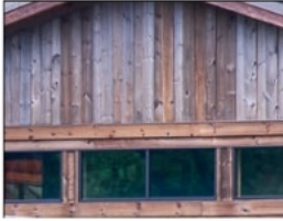
Unpainted board and batten siding
