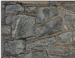
Rough cut granite with irregular courses
