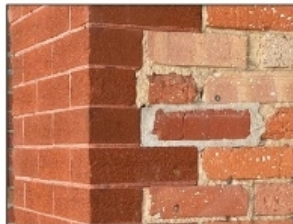
Red brick with flush mortar is used as veneer
