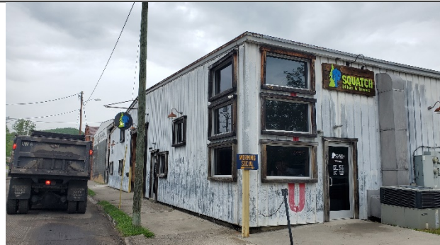
Multi-tenant converted warehouse
