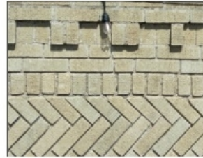
Herringbone brick pattern in parapet
