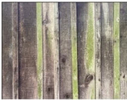
Unpainted board and batten siding
