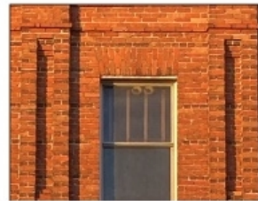
Red brick wall with structural pilaster and flat arch
