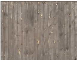
Unpainted board and batten siding
