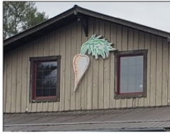
Painted board and batten siding
