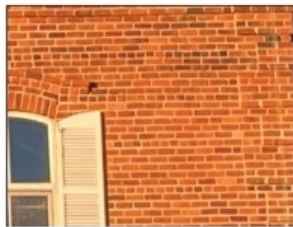
Red brick with common bond and quoining
