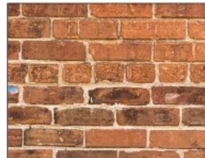
Red brick with common bond and concave mortar
