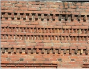
Decorative brickwork in the parapet
