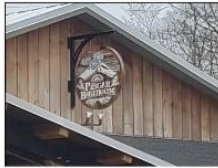
Unpainted vertical plank siding
