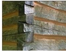
Unpainted wood logs with visible clay chinking
