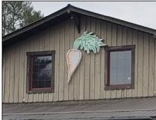
Painted board and batten siding
