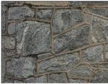
Rough cut granite with irregular courses
