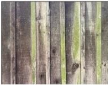
Unpainted board and batten siding
