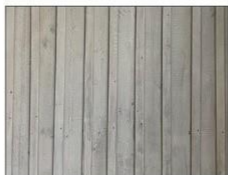
Painted board and batten wood siding
