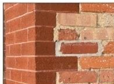
Red brick with flush mortar is used as veneer
