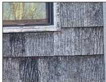
Unpainted rustic wood siding
