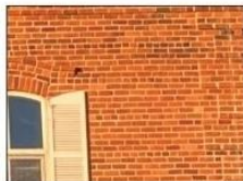
Red brick with common bond and quoining
