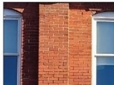
Red brick wall with a structural pilaster
