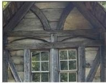
Unpainted wood plank siding with half-timbering
