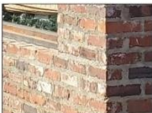
Multi-color brick with extruded mortar
