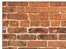
Red brick with common bond and concave mortar
