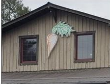
Painted board and batten siding
