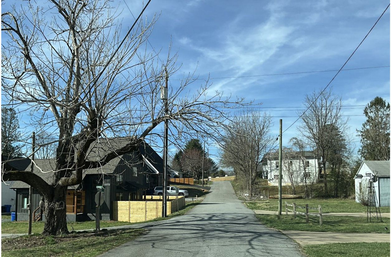
Pic 3- Street view of slope on Turnpike Rd, 188 Ashworth on left side of pic.
