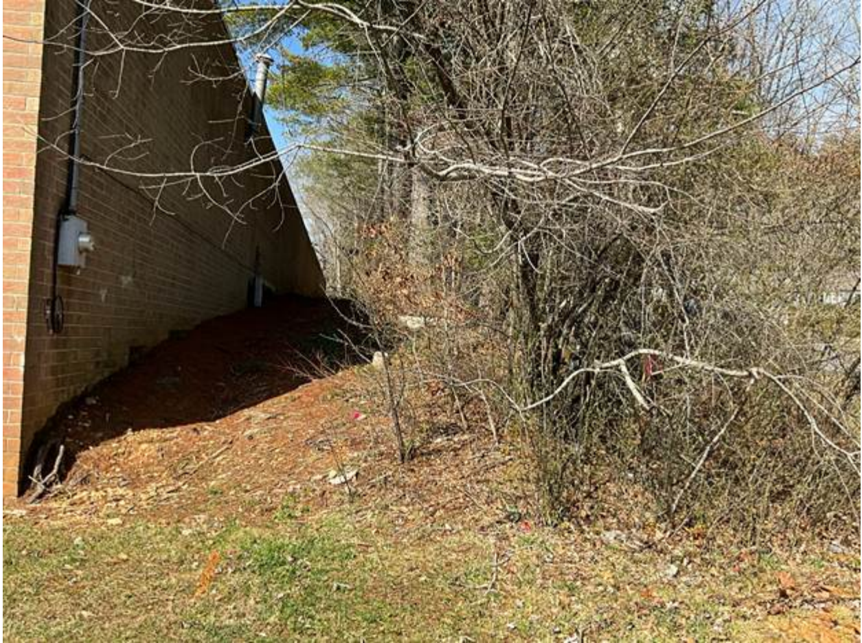
(View from Burrell Ave looking at the existing side yard, vegetation and existing North wall)
