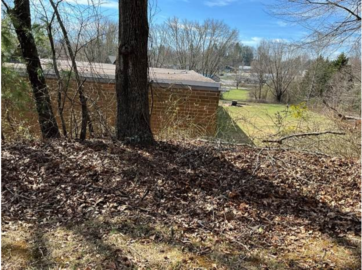
(View from Peace Ave of the North wall and NW corner of the existing building)
