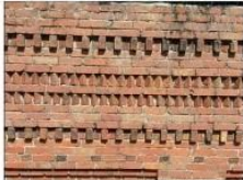
Decorative brickwork in the parapet
