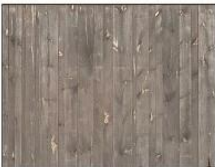
Unpainted board and batten siding
