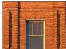
Red brick wall with structural pilaster and flat arch
