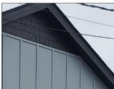
Painted fiber cement board and batten siding
