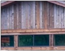
Unpainted board and batten siding
