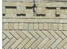
Herringbone brick pattern in parapet
