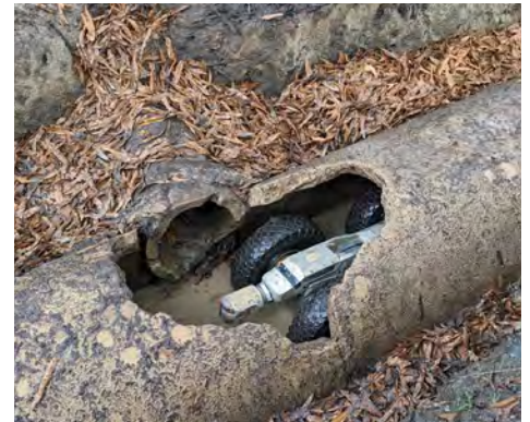
CCTV Storm Pipe Inspections
