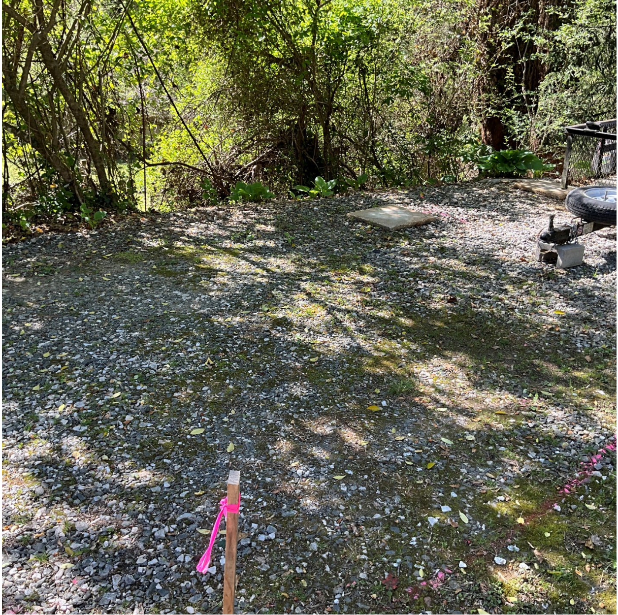
Visible topography changes on left of existing driveway
