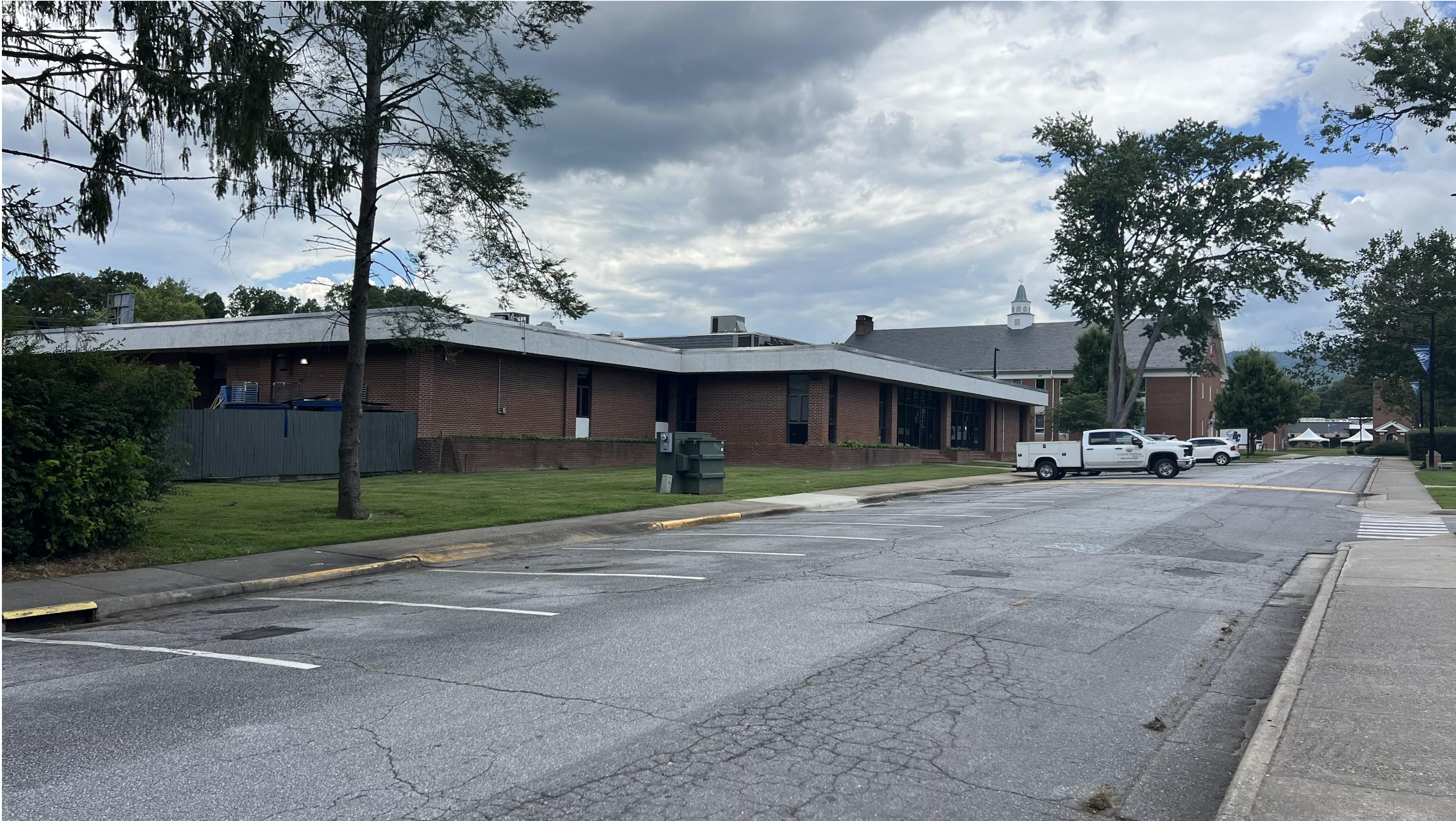
1 - EXISTING VIEW CAMPUS DRIVE NORTHWEST CORNER
