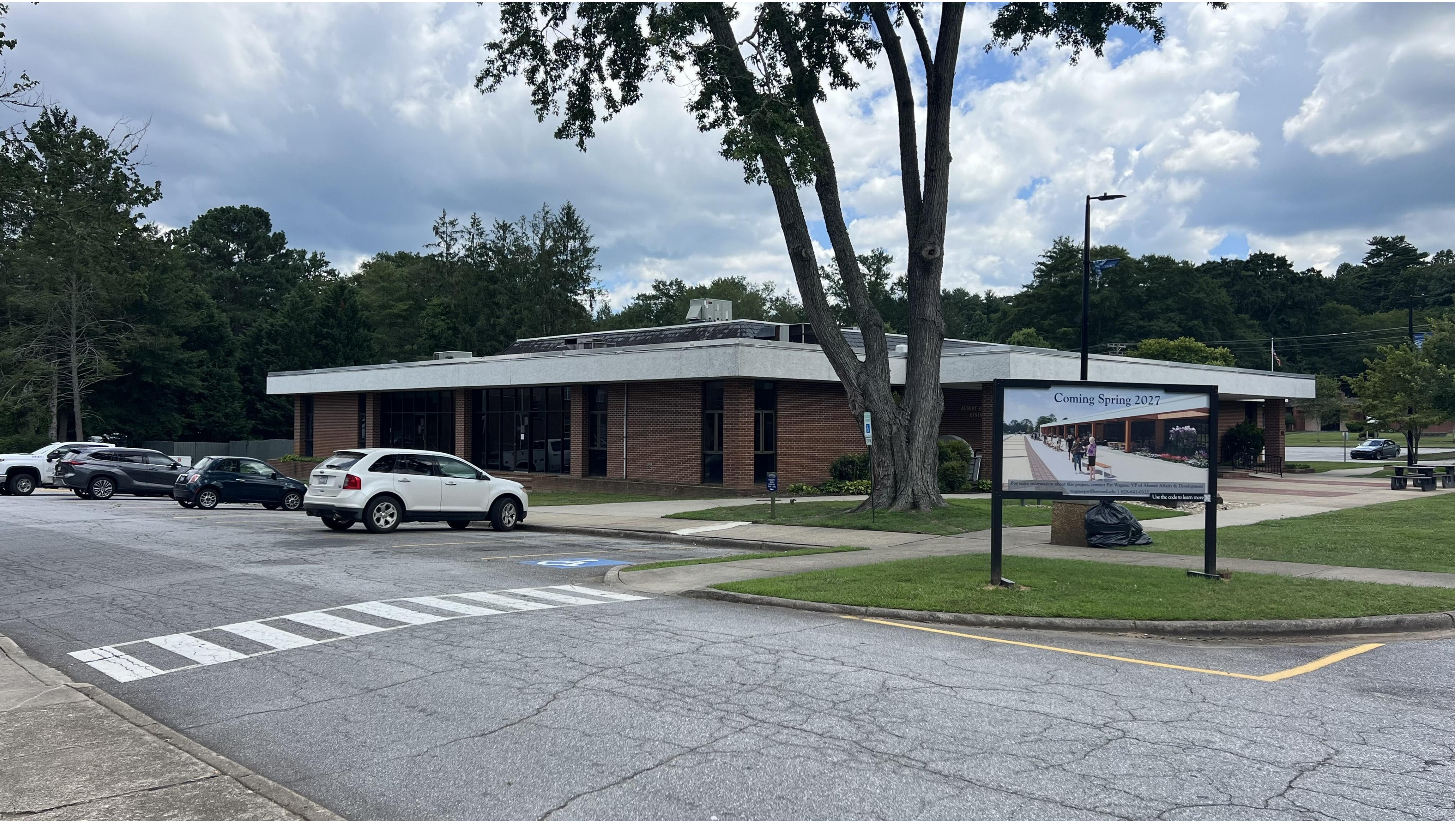
2 - EXISTING VIEW CAMPUS DRIVE NORTHWEST CORNER
