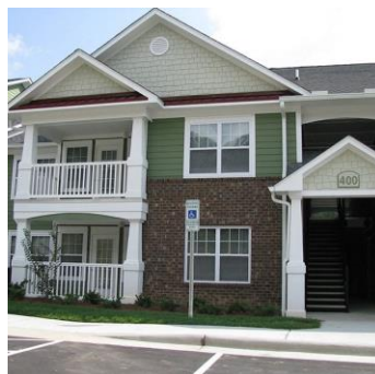
Broad River Terrace Brevard, NC (60 Units; 2011)
