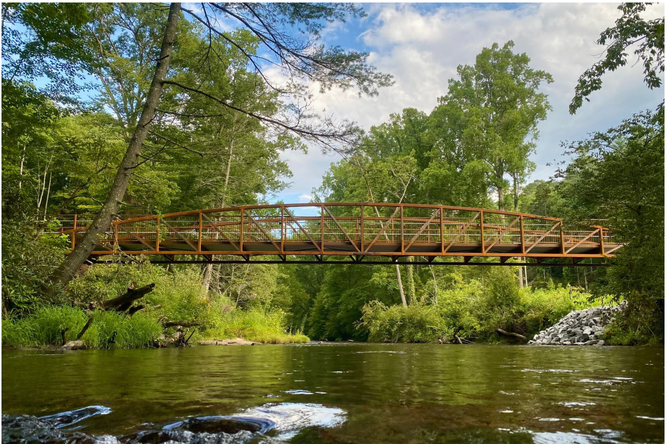
Pedestrian bridge over Davidson River. Image Source: City of Brevard
