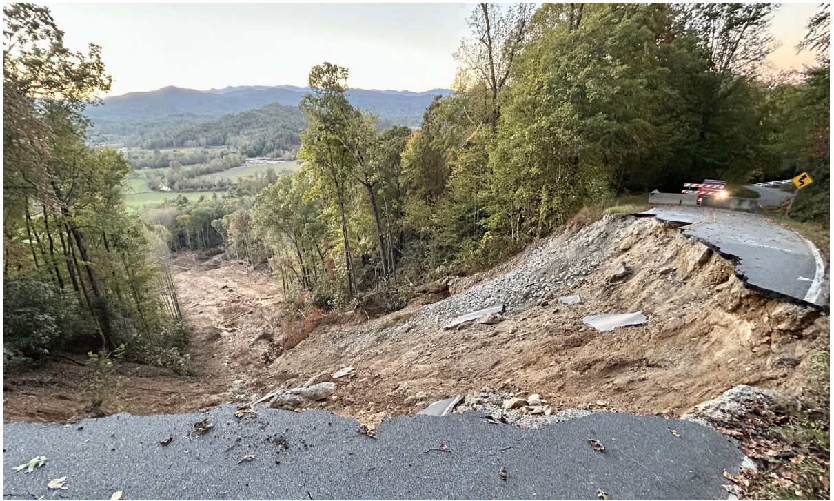
Landslide on Becky Mountain Road outside of Brevard following Tropical Storm Helene. Image Source: City of Brevard
