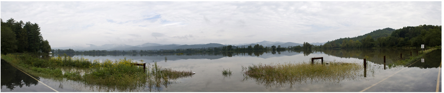
Panoramic view of a flooded Wilson Road. Image Source: City of Brevard.
