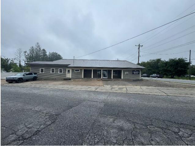
Site along Oakdale Street, from south.
