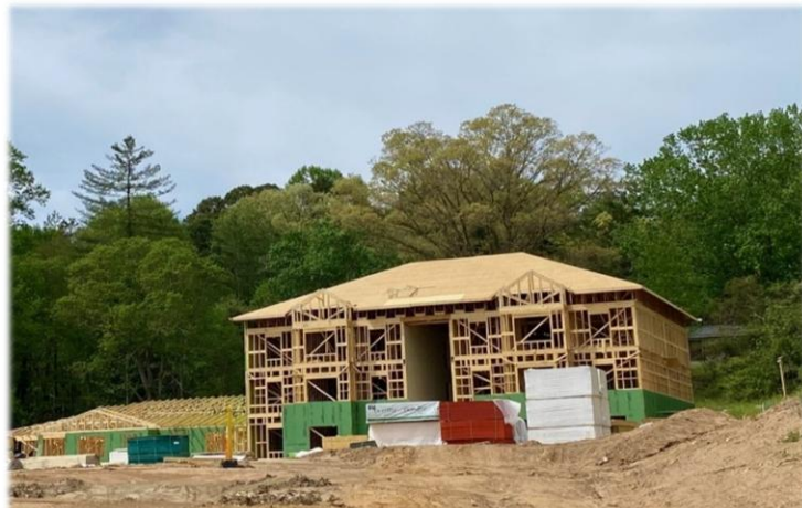
Funded partially by a $1.1M loan from the City, 48-units of low-to-moderate income housing is under construction off Asheville Highway. The units will serve families making below 80% of area median income.
