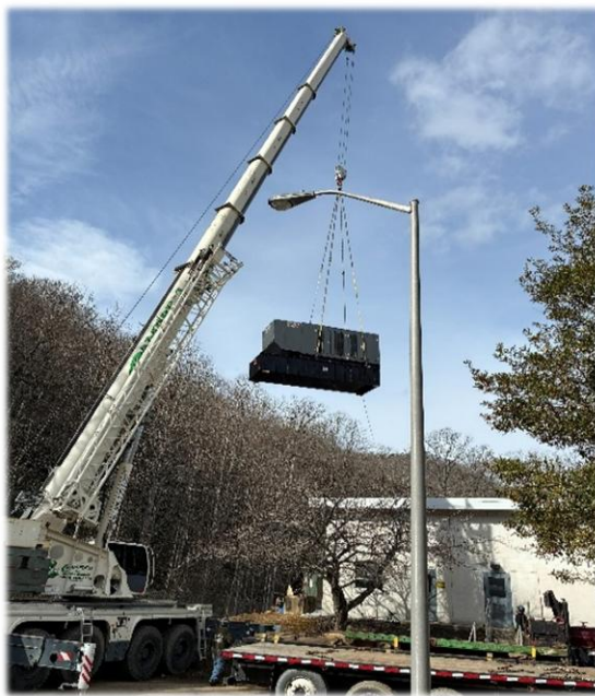
A new generator is installed at Brevard's water treatment plant.
