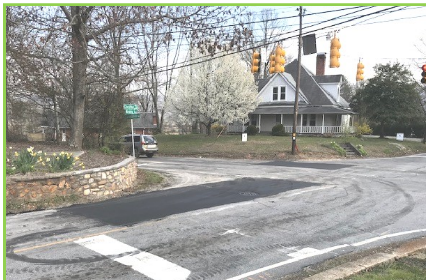
Old Highway 64 utility cut patching by JLS Paving, LLC.
