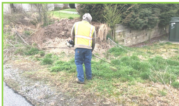
Trimming weeds at the Bedford Place Lift Station.
