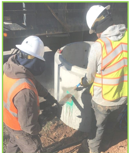
Cutting tap in new manhole for future construction.
