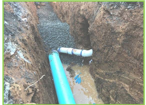
4" commercial sewer tap installation on W. Main Street.
