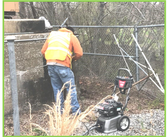
Completed exterior pressure washing of old lift station.
