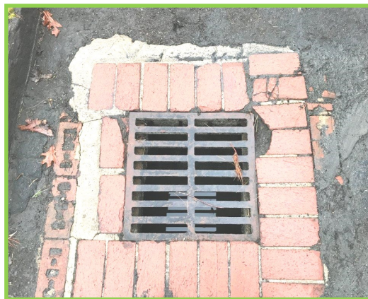
E. Main Street storm drain inspection.
