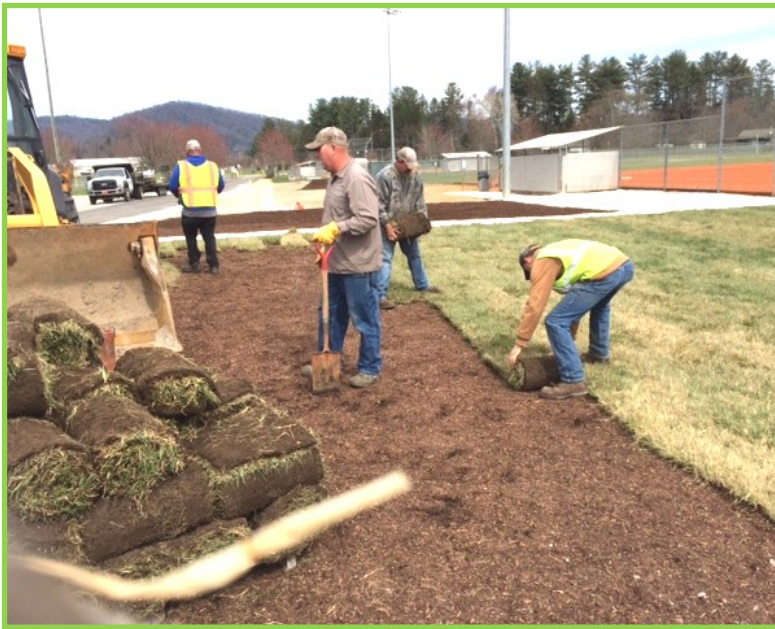
Additional sod installation at the Sports Complex ball fields.
