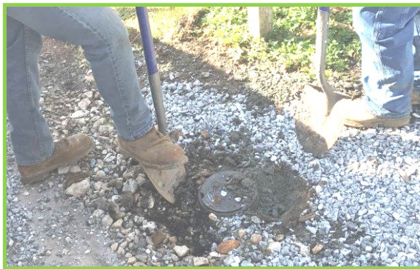
Carolina Avenue sewer cleanout valve box removal.
