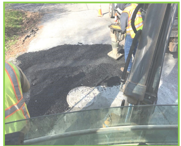
Hawthorne Drive site restoration.
