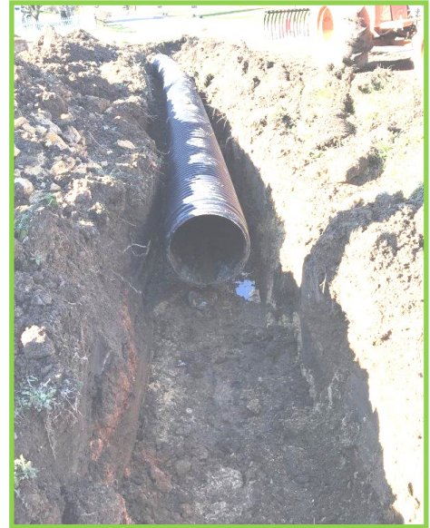
Cashiers Valley Road storm drain installation.
