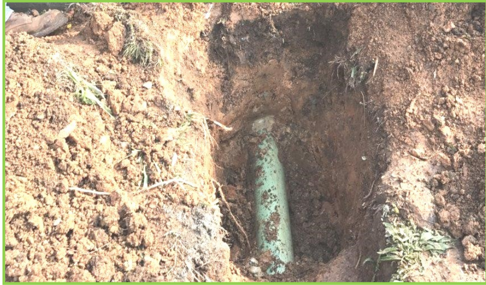
Excavated 6" sewer service line from the garage wash pit.
