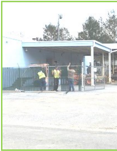
Installing Operations Center privacy slats.
