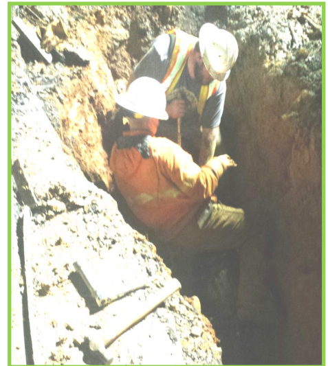
Jordan Street water main relocation.
