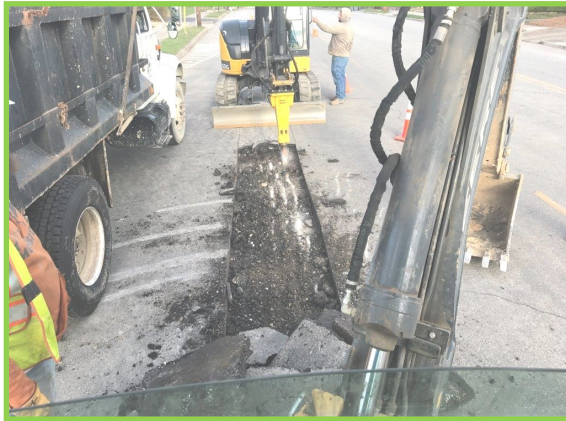
W. Main Street asphalt removal.
