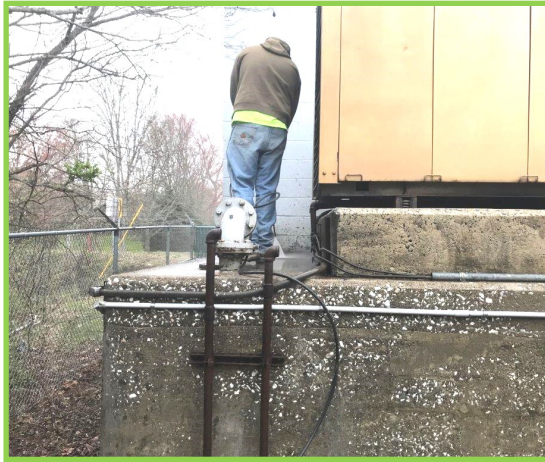
Neely Road Lift Station pressure washing.
