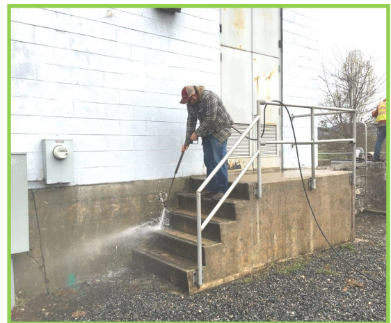
Pressure washing the exterior of the old Neely Road Facility.
