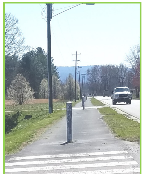
Eastatoe Trail trail maintenance and weed control.
