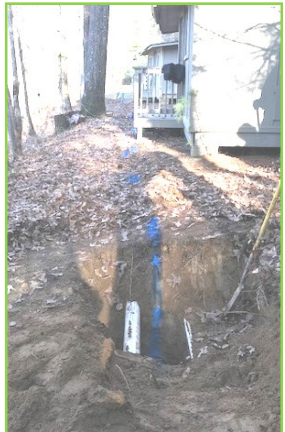
Brevard Music Center water line locate.
