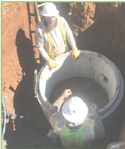
Leveling new Elliott Road manhole base.
