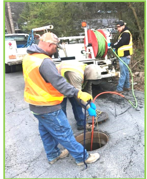
James Street 8" service line cleaning.
