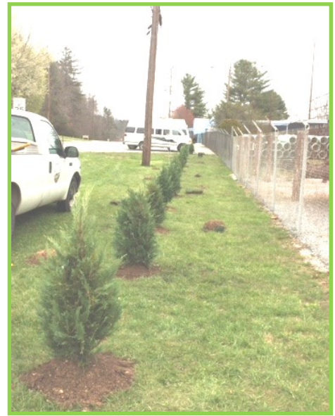
Leland Cypress tree installation.
