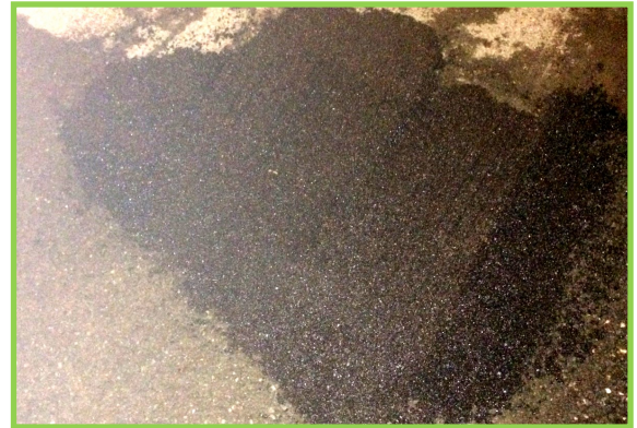
Country Club Road pothole repair.
