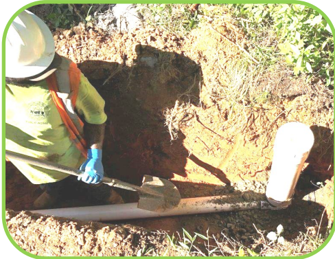
Tinsley Road sewer service line and clean check replacement.
