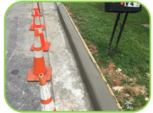
Thomas Street curb installation.
