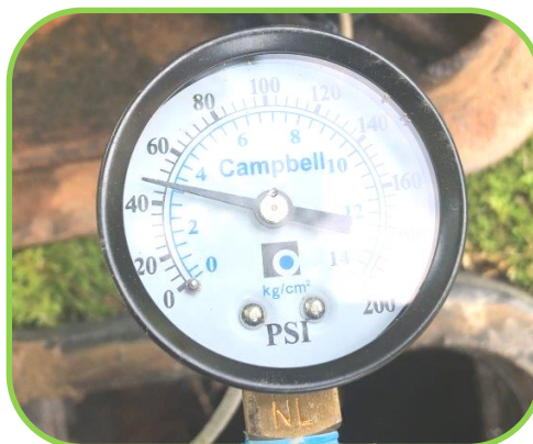
Gauge used to inspect Ridgetop Circle pressure at water meter.
