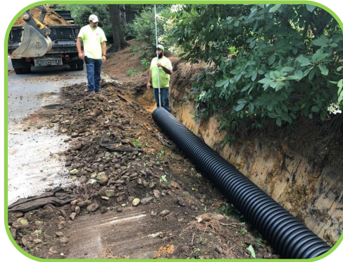
Ensuring grade for Lakeview Avenue storm drain installation.
