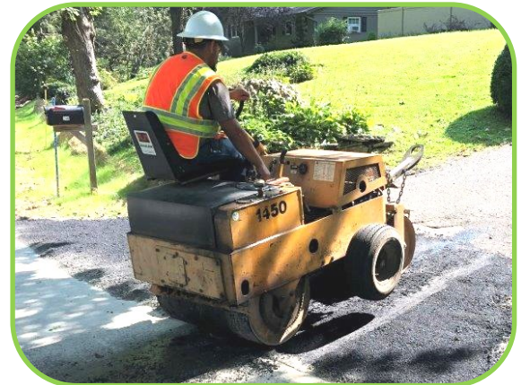
Asphalt roller compacting hot mix on Lakeview Avenue utility cut.
