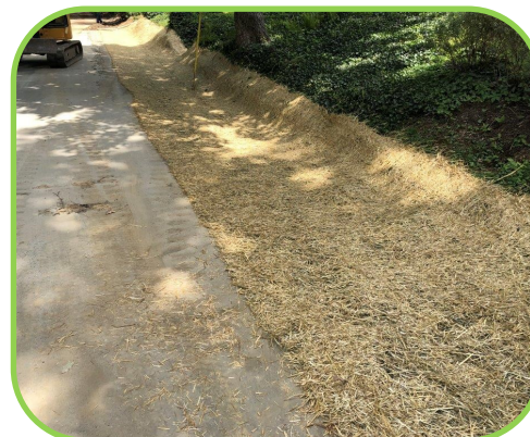
Straw matting placed to stabilize and prevent erosion.
