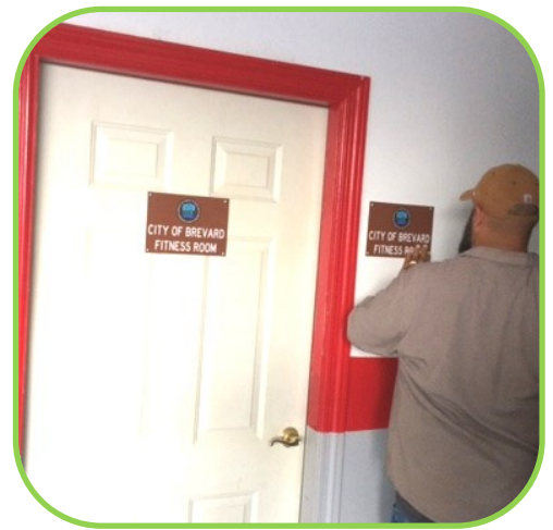
Fitness Room signs erected.
