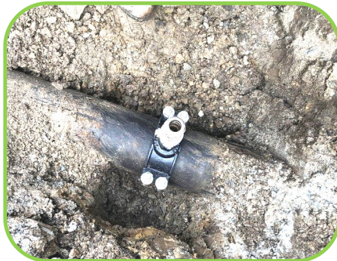
1" Corporation on 6" water main prior to tap.
