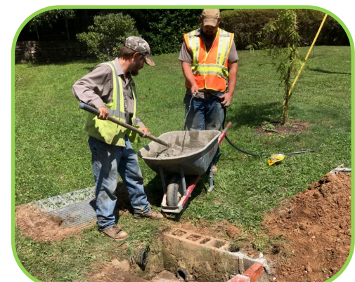
Concrete mixture prepared for Hilt Street junction box.
