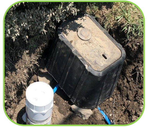
Relocated Whitmire Street water meter box.
