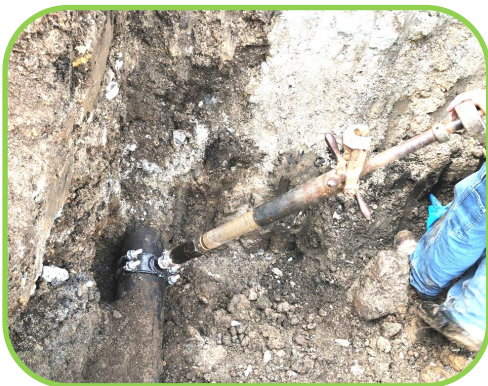
Tapping machine connected to complete Depot water tap.
