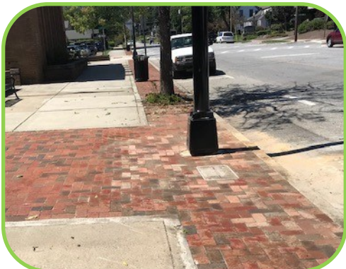
W. Main Street sidewalk restoration.
