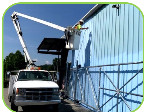
Spray painting exterior of Public Works Building.
