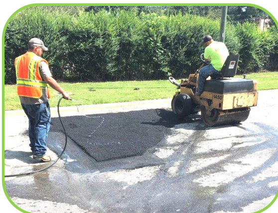
Excelsior Drive utility cut patching.
