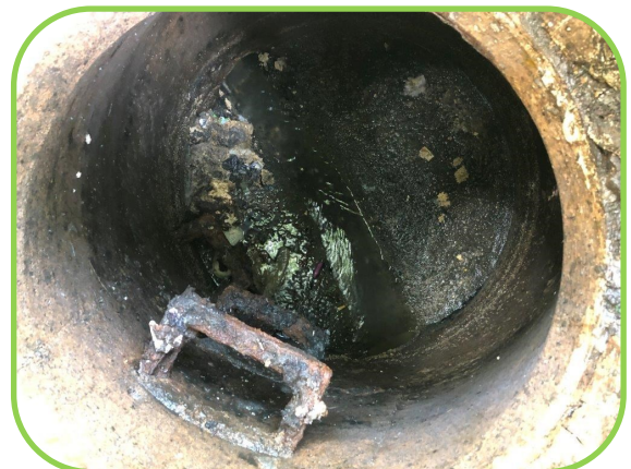
Manhole #LS-070 with adequate flow following grease removal.
