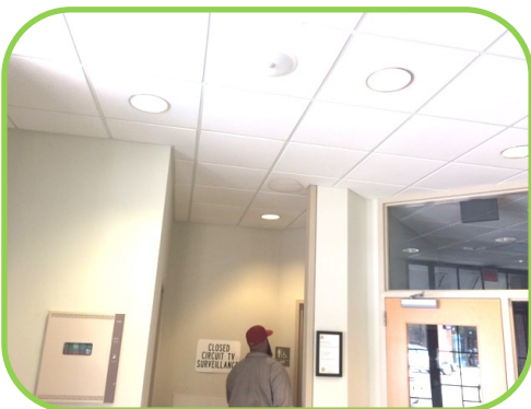
Facility light fixtures inspected in Council Chambers lobby area.
