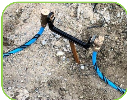
Service line and yoke bar connected pending water meter installation.
