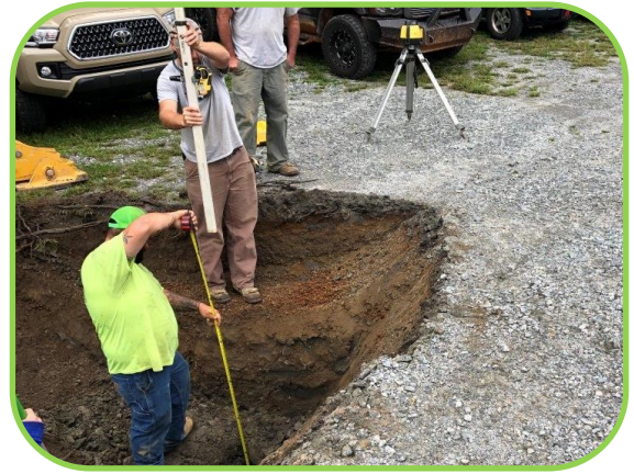
Railroad Avenue assistance with grade for storm drain installation.
