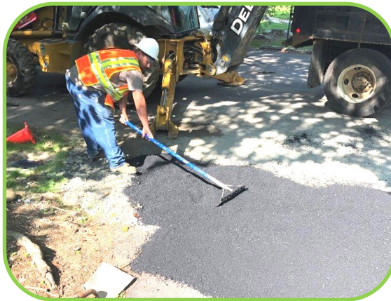
Leveling hot asphalt mix into Lakeview Avenue utility cut.
