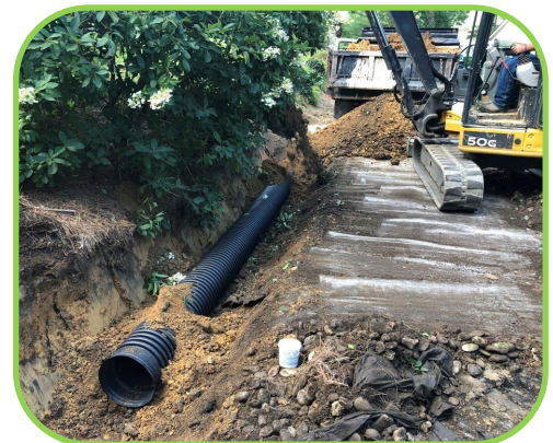
Backfilling to secure pipe installation.
