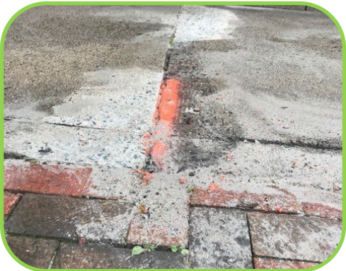
W. Main Street sidewalk edge leveled to eliminate trip hazard.
