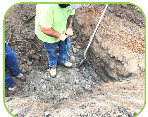
Probing to confirm location and depth of 8" Whitmire Street sewer main.
