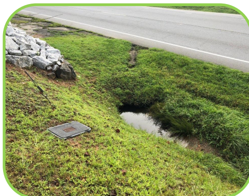
Asheville Highway drain inspection.
