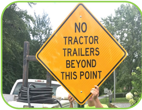
Big Bend Road sign installation.
