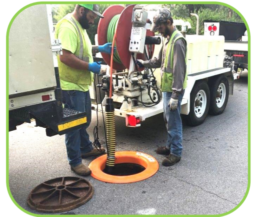
Onyx Lane sewer line cleaning within Brushy Creek Basin.
