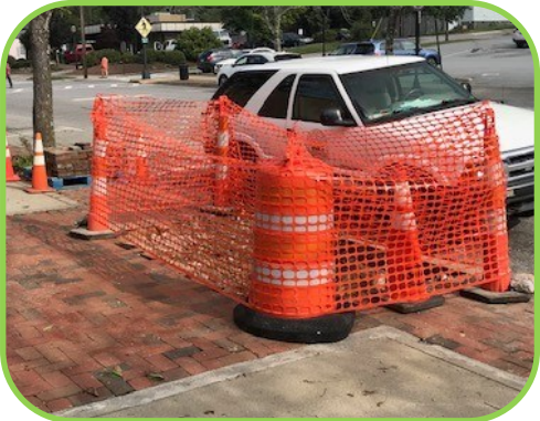
W. Main Street preparation for utility pole replacement.
