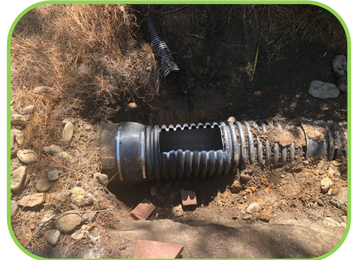
Pipe opening cut for basin access.
