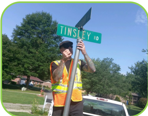
Resada Drive and Tinsley Road sign repair.
