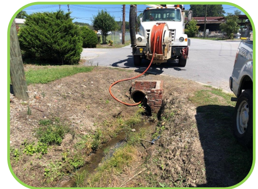
Railroad Avenue dye testing to verify drain flow direction.
