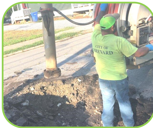
Hydro-excavation to deteriorated clay sewer taps on Whitmire Street.
