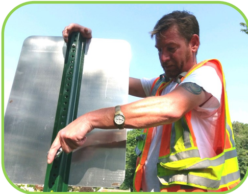
N. Johnson Street speed limit sign installation.
