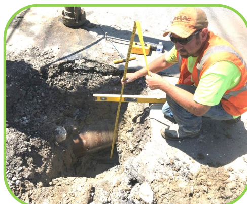
Depth confirmation of Railroad Avenue 6" water main.
