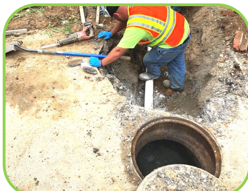
Connecting 4" service line pipe into manhole #JB-084.
