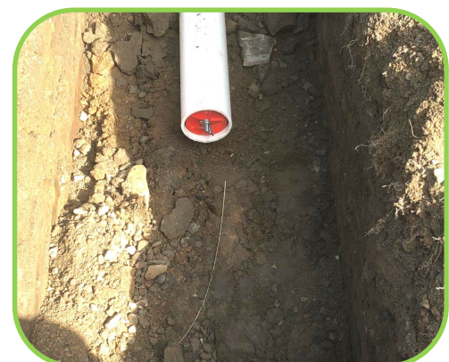
4" Sewer service line plugged until contractor is ready to connect.
