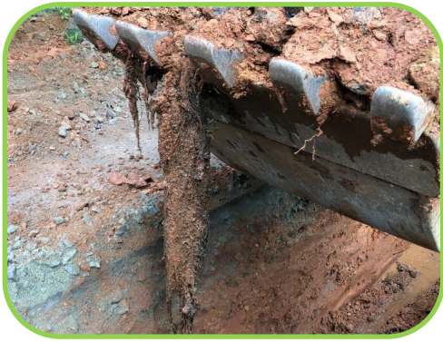
Tree roots removed from Tinsley Road service line.
