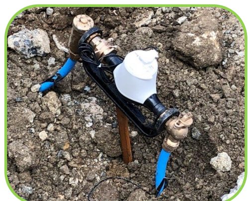
1" Water meter installed into yoke bar to serve Depot Building.
