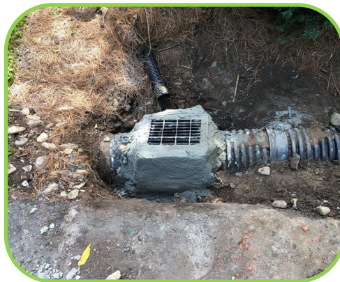
Catch basin installed on drain pipe opening.
