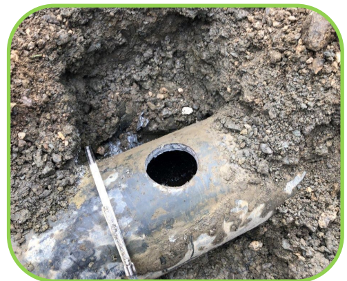
Railroad Avenue Depot 4" tap drilled into sewer main.
